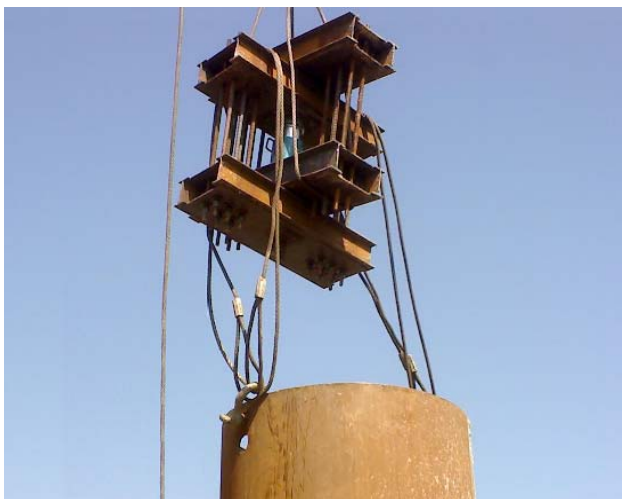
Fig. 3 Imposing tension force to pile
