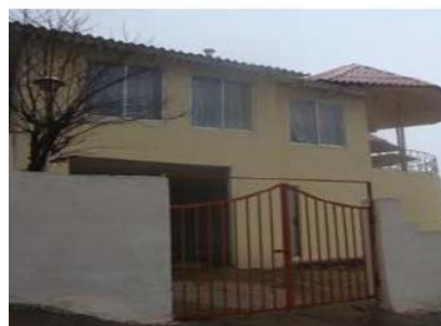
Fig. 14 New construction in staircase structure of Masouleh
