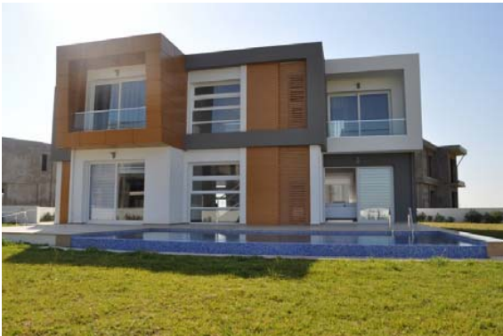
Fig. 4 Use of cumba with the new interpretation in Famagusta modern houses (Photo by author)
