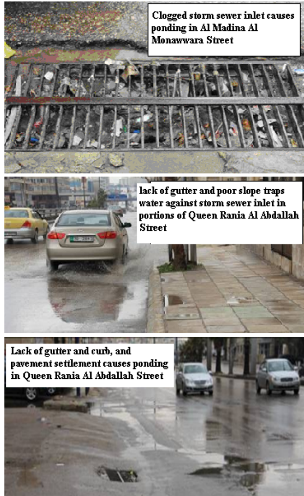
Fig. 3 (b) Example Problems of the roadway drainage systems in Site 1
