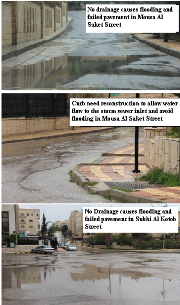
Fig. 3 (a) Example Problems of the roadway drainage systems in Site 1
