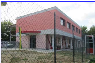
Fig. 20 View of the building after the completion of the retrofit and architectural renovation works
