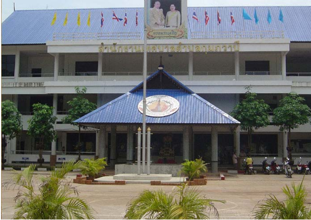
Fig. 2 The Municipal Office of sub-district Kumphawapi
