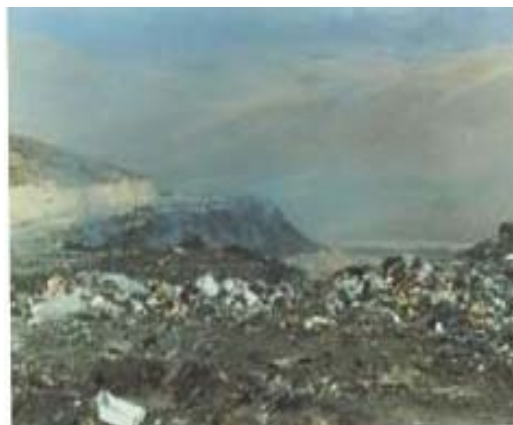
Fig. 7 View of uncontrolled dumping of wastes in landfill site
