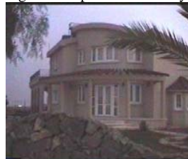
Fig. 7 Villa type house in Tuzla
