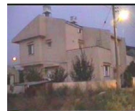
Fig. 12 Disconnected buildings in Tuzla
