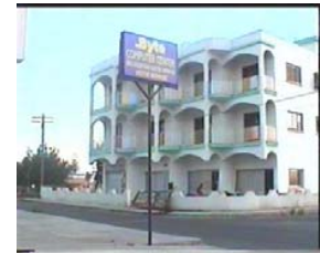
Fig. 6 New apt. blocks in Baykal
