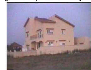
Fig. 8 Villa type house in Tuzla
