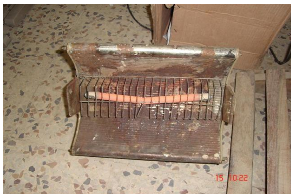
Fig. 15 Unsafe electric heaters being used at retail outlet
