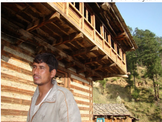
Fig. 5 Traditional 'Kath-khuni' wall construction with timber & stone
