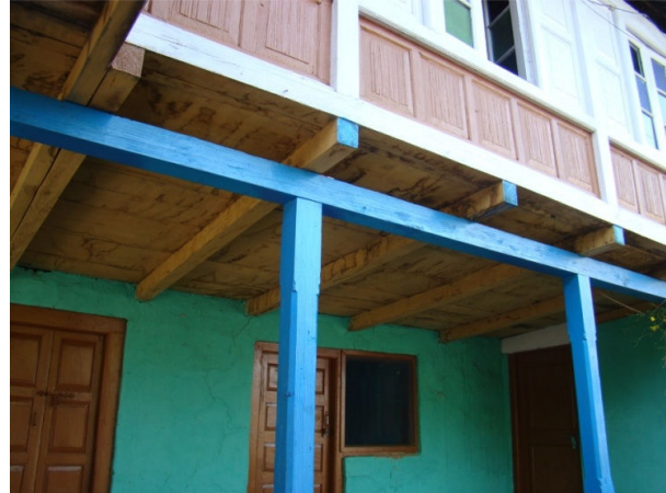
Fig. 6 Timber flooring and cantilevered balcony
