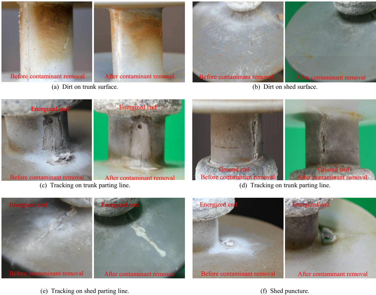
Fig. 5 Surface damage of tested specimens.
