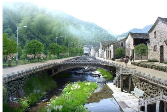
Fig. 8 Riverbank landscape remediation and facilities enhancement
