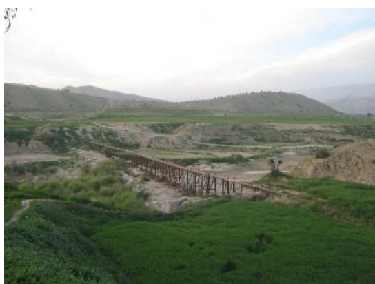
Fig. 6 The oil pipe line is located on the upstream of Kowsadam basin next to Choram , station 4
