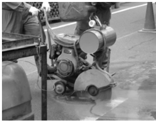
Fig. 1 A road cutter is cutting the road
