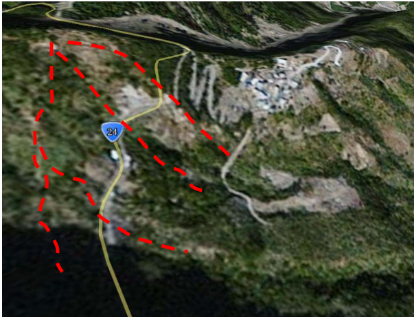
Fig. 13 Collapse Zone of Linear Structure (Google Earth)
