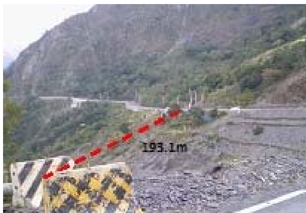
Fig. 1 Location of slope collapse and sliding
