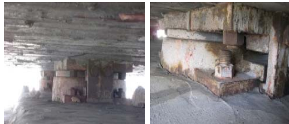
Fig. 8 Bearing steel plate
