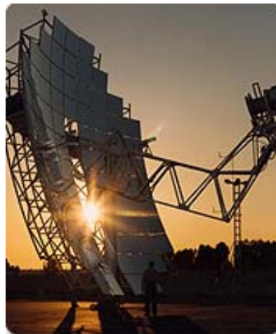
Fig. 1 Parabolic dish concentrator [5]
