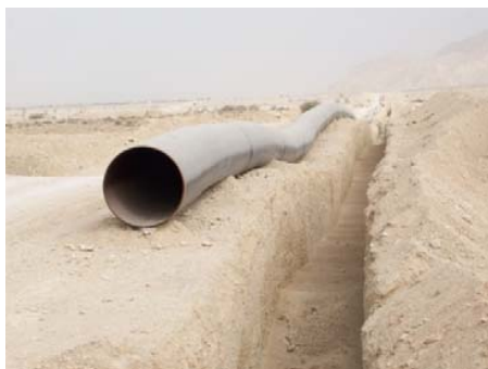
Fig. 3 36 inches Assalouyeh-Bandarabbas gas pipeline project
