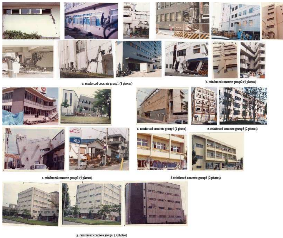
Fig. 2 Damaged photographs of frame structure
