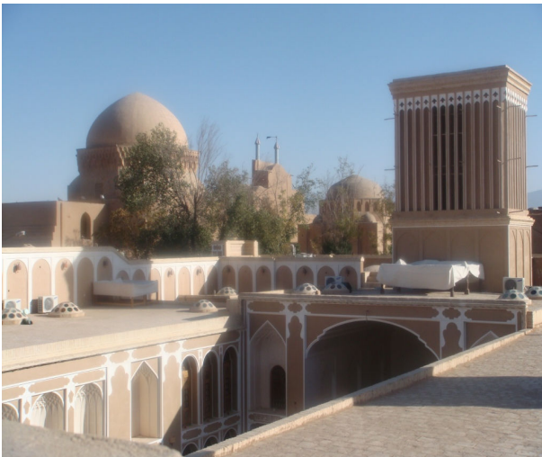
Fig. 1 The way of yard position in the centre and using the air hole (Yazd, Iran)
