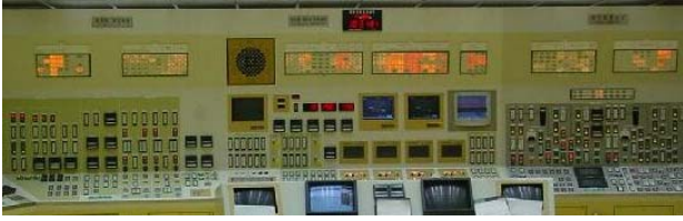
Fig. 7 Alarm windows in the conventional control rooms
