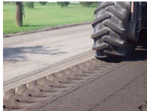
Fig. 2 Blending fly ash with pulverized base material
