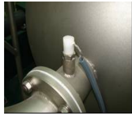
Fig. 9 PT100 Temperature sensor
