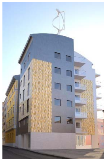
Fig. 1 Rendering of the Panorama Giustinelli Building, showing also the selected position for the placement of the WECS
