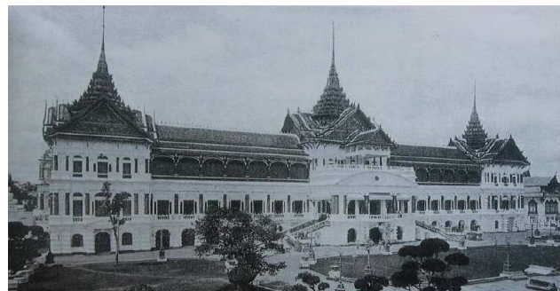
Fig. 12 Architecture of Chakri Maha Prasart Throne Hall Before restoration
