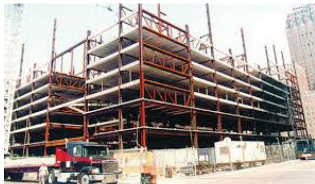
Fig. 3 Staggered truss system
