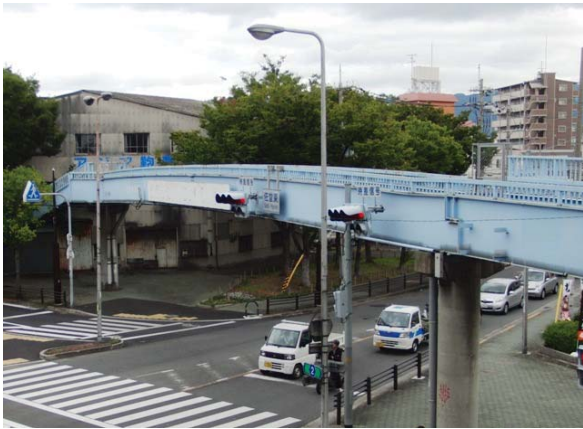
Fig. 1 Footbridge being tested
