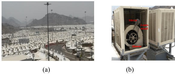
Fig. 4 (a) Mina Valley pilgrims' tents (b) roof-top evaporative cooler unit
