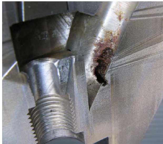
Fig. 9 Cavity found at defect location
