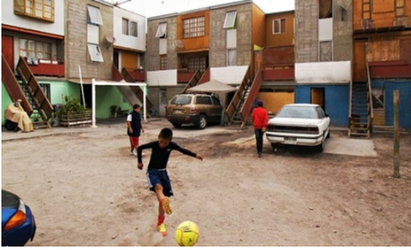
Fig. 6 Quinta Monroy after the users' intervention [31]
