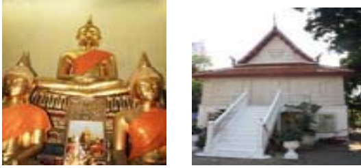
Fig. 15 Phra Samput Wattanopat (left) and King Rama IV's monk residence (right) in Wat Rajadhiva Vihara which were restored by King Rama IX
