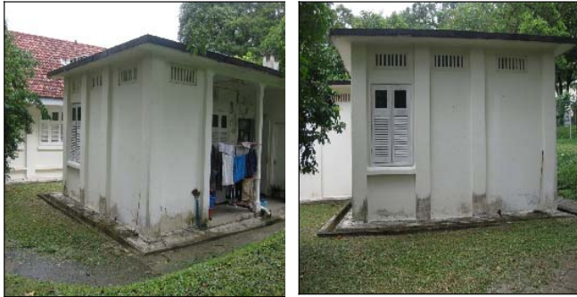
Fig.1 Test room located at the back of the main building
