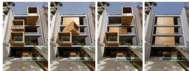
Fig. 2 Rotating rooms- Sharifi-ha house [7]
