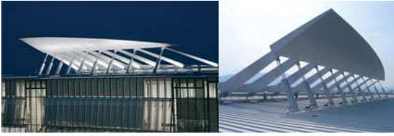
Fig. 4 The Transformable roof of the new Merck Serono Headquarter
