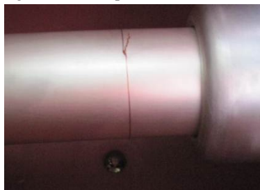
(a) Tip on the high-voltage conductive pole
