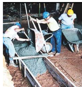
Fig. 1 Conventional method to mix concrete and to cast it on site
