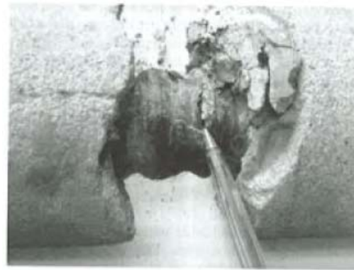
Fig. 2 Rupture of the DCP bolt plastic sheath after [1]
