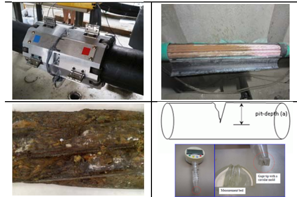
Fig. 1 Inspection procedure for corroded tendon
