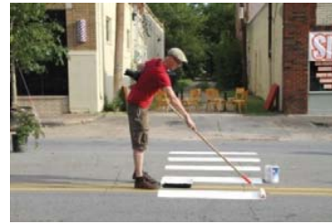
Fig. 3 Better Block Volunteer create new crossing lines in Oak Cliff, USA [16]
