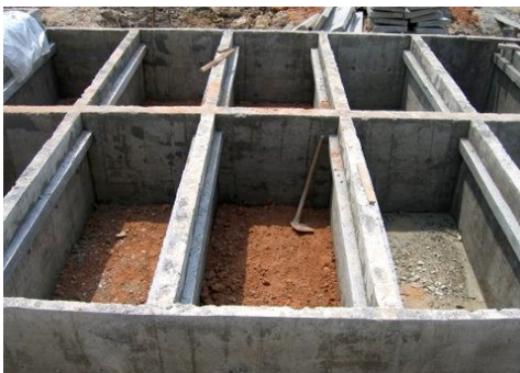
Fig. 20 Picture shows the use of pre-cast concrete at Subang Lutheran Garden (Lei Wei Min)
