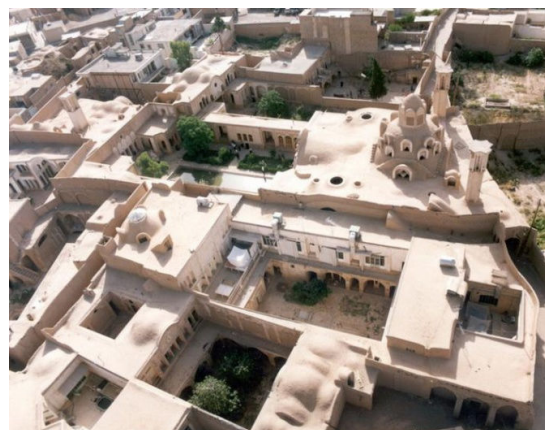
Fig. 2 North and South Parts of a Borujerdiha House in Yazd City; Photo by Iran News Agency [20]
