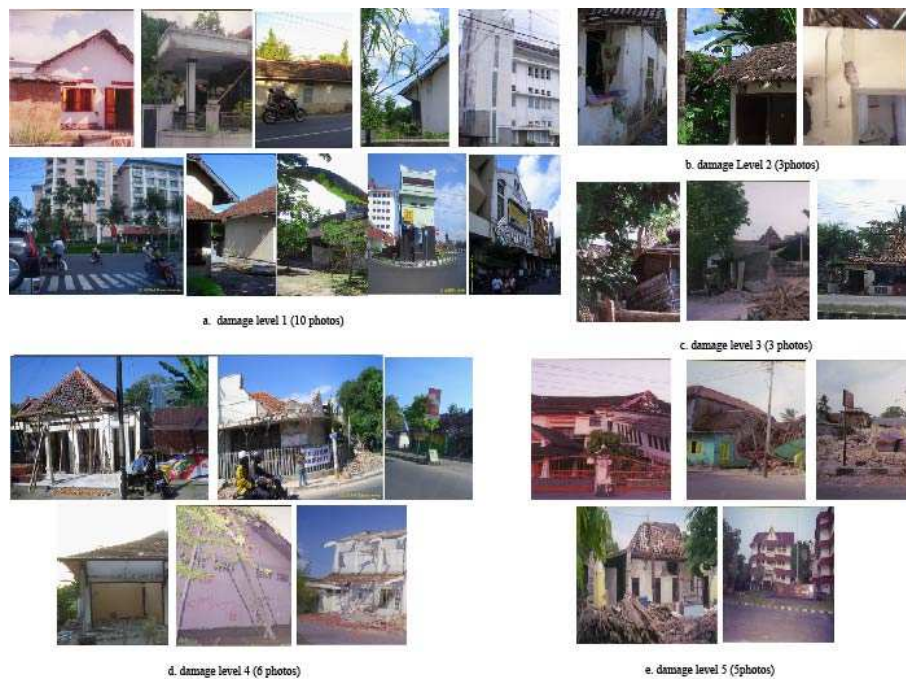
Fig. 1 Damaged photographs of masonry structure
