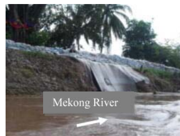
Fig. 3 Sheet-Flood erosion control work situation*
