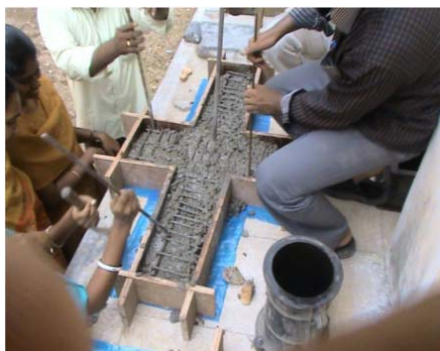
Fig. 9 Casting of beam column joint
