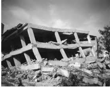
Fig. 5 Beam column Joint failure
