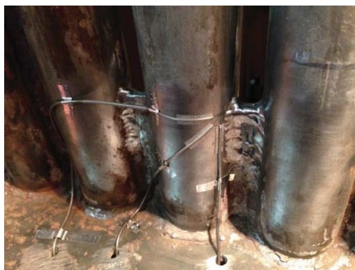
Fig. 3 Strain gage installation on boiler tubes
