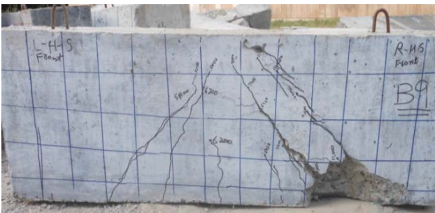
Fig. 9 457mm (18in) deep beam crack pattern
