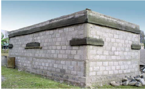
Fig. 7 (a) Roof band beam and wall L-stitches
