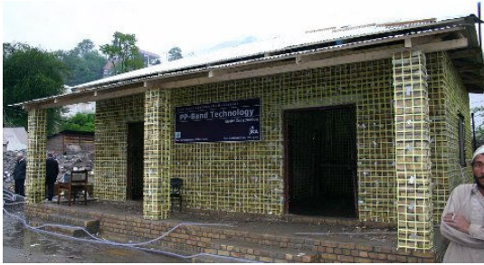
Fig. 7 (b) Polypropylene band reinforcing
