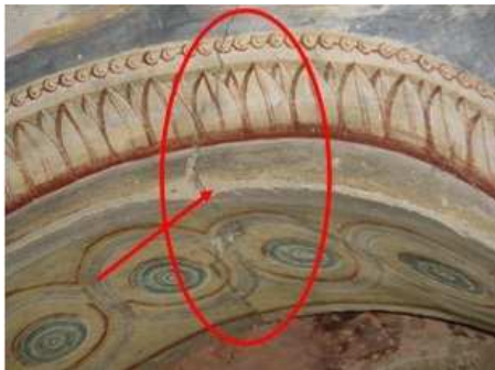
Fig. 16 Cracks at arches
