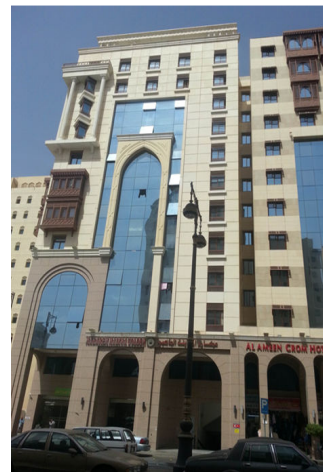
Fig. 3 Front view of the case study building in Madinah
