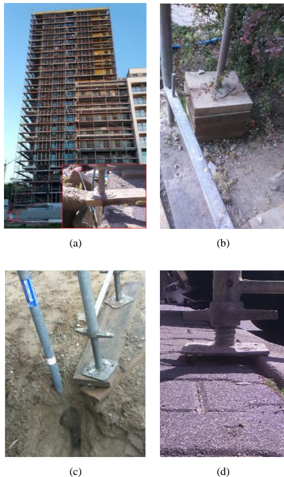
Fig. 2 Errors in scaffolding supports; (a) strained mudsill, (b) multi-level wooden mudsills, (c) unstable substrate, (d) base jack without support
